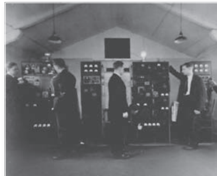
Training on communication equipment.
