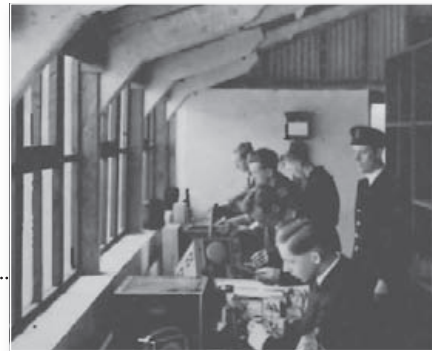
Radar training at HMS Mercury.
